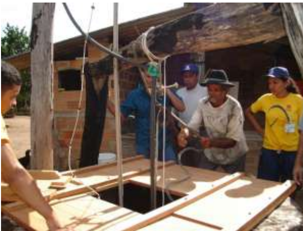
Figure 3: Installing and Testing the Well Cover
