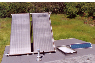
PV pumped solar hot water collector for drain-back hot water system.
