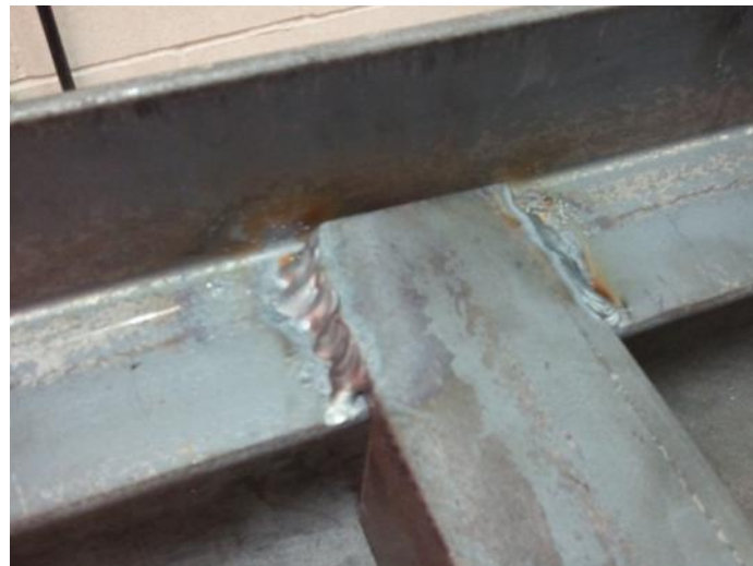
Figure 19: Center support welds
